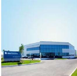
More than doubling production capacity: Aker Solutions' new 90 000 square foot manufacturing facility in Pickering, Ontario, Canada.
